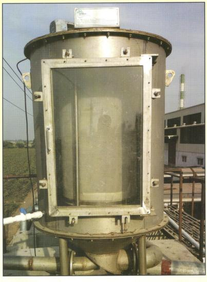
Raw water enter the system under pressure of about 1Kg/Cm² (14.2psi)
